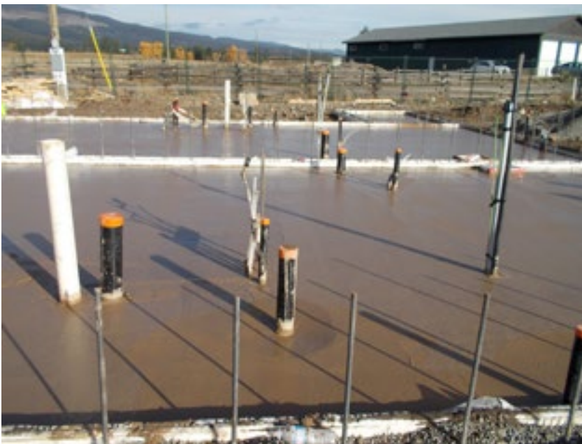
Radiant concrete flooring poured in the new duplexes under construction.
