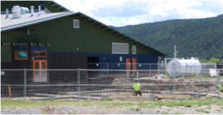
Construction happening at the School.
